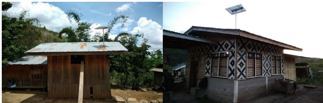
Diagram 7: Roof-through Pole mounted installations on GI roofs
