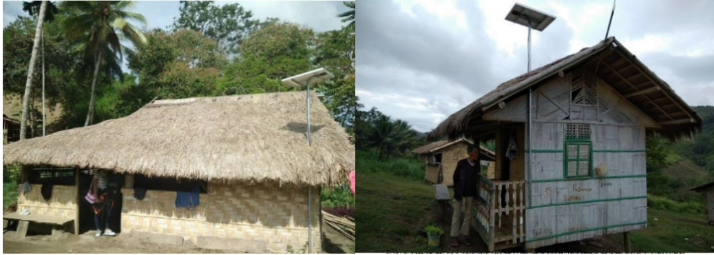
Diagram 8: Roof-through Pole mounted installations on thatched roof
