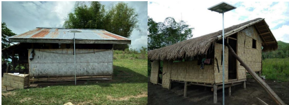
Sample Roof-side Pole mounted installation
